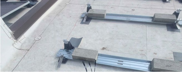
Mounting System Anchoring: Photo showing flashing techniques utilized for applicable flat roof projects.
