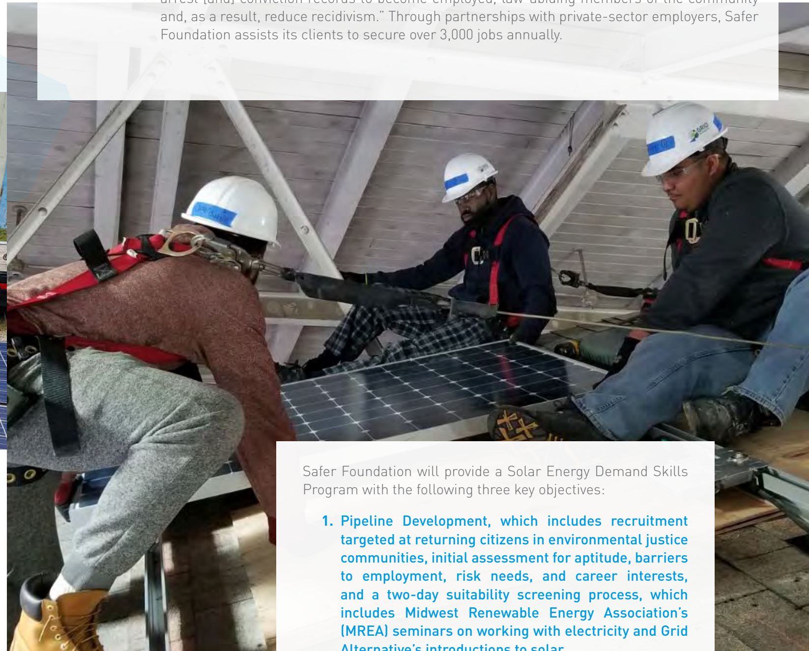
Solar Boot Camp – solar panel installation
